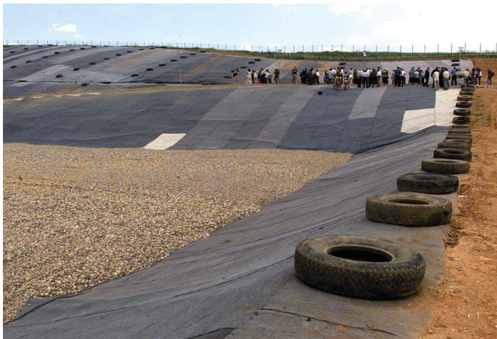
Proper linings help to prevent dangerous substances from escaping.
